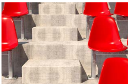
Stadium seating anchoring
