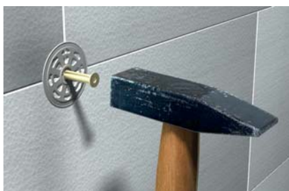
Flush hammerset installation
